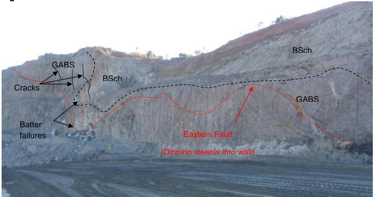
To provide long term stability a cutback is required to lay the slope back to a flatter angle, refer to Figure 2. This requires the new crest to be behind the current PEPR boundary
